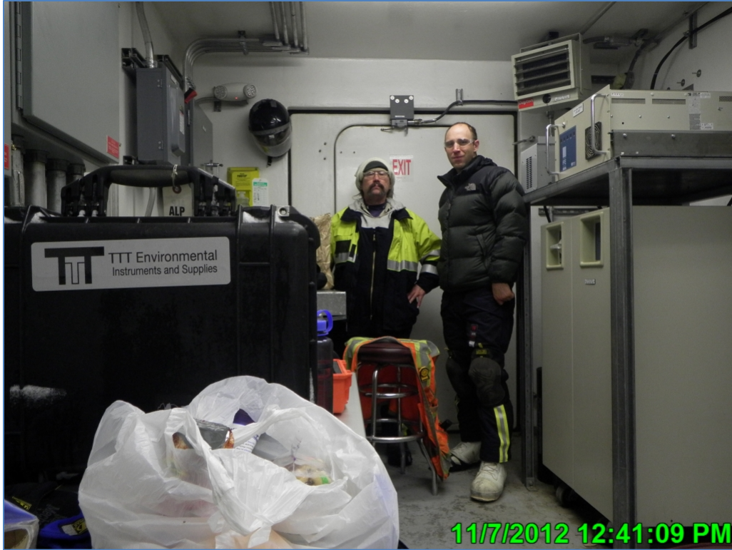
Photo B.7: HDD warm up shack; November 7, 2012
