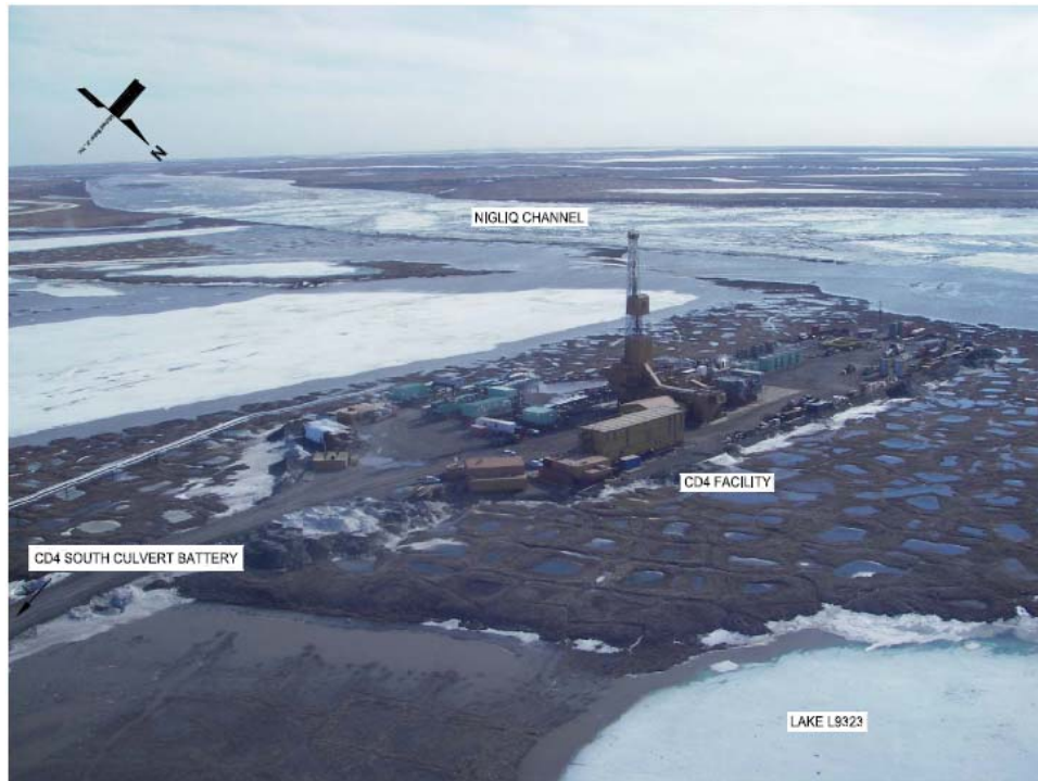
Figure 4: South culvert battery (out of picture) flow entering Lake L9323(June 4, 2007)
