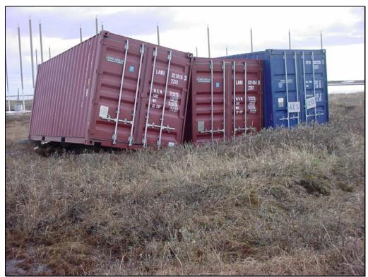
Photo 14 – HDD crossing, east bank. ACS spill response container jacking due to uneven settling of on-grade support beams. June 17, 2004.
