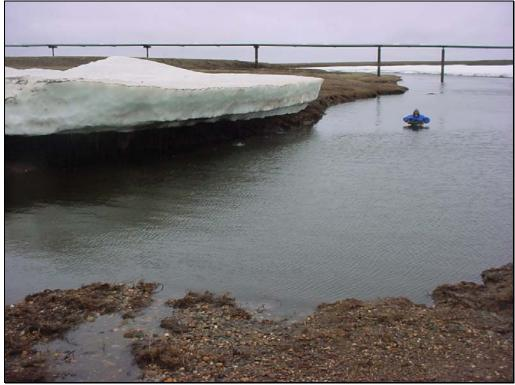
Photo 18 – Kachemach River, left bank looking downstream. Water depth increased rapidly within the scour hole at the ice road route. June 18, 2004.
