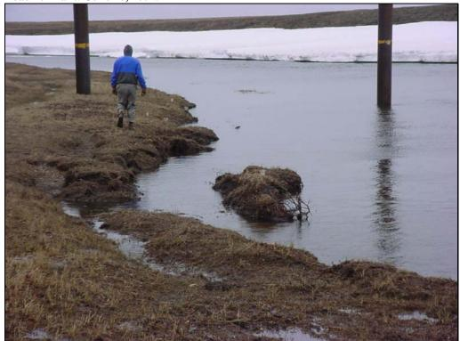
Photo 20 – Kachemach River. Localized slumping on left bank was documented in 2003 investigation. 2004 bank deterioration in this area was minimal. June 18, 2004.
