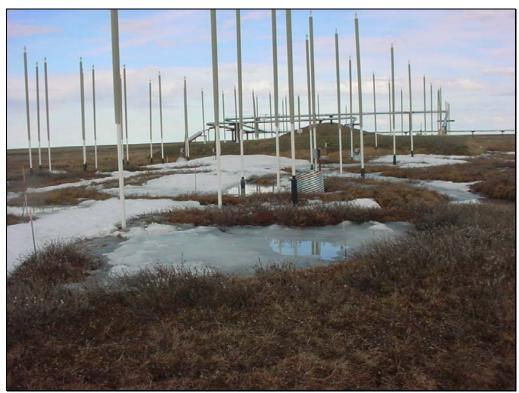
Photo 12 – HDD crossing, east bank. Thermosiphons along south pipeline alignment, no settling or jacking noted. June 17, 2004.
