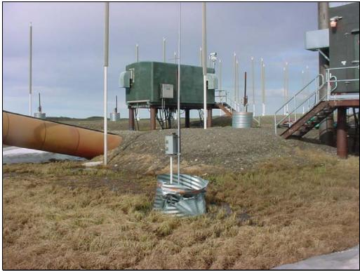
Photo 8 – HDD crossing, west bank. No gravel deterioration on pad. Note damaged protective CMP at thermistor string location. June 17, 2004.
