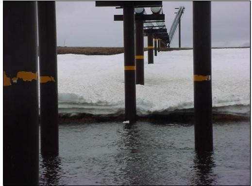
Photo 22 – Kachemach River. All VSMs and HSMs appeared straight and level. June 18, 2004.
