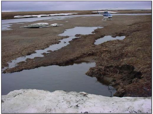
Photo 19 – Kachemach River, left bank looking upstream. Minimal scour on gravel bar upstream from the scour hole suggests that scour was localized. Note minor bank sluffing just upstream from the ice road remnant. June 18, 2004.
