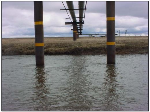
Photo 27 – Miluveach River. The right bank appeared stable and well vegetated. All VSMs and HSMs appeared straight and level. June 18, 2004.
