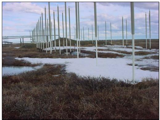
Photo 13 – HDD crossing, east bank. Thermosiphons along north pipeline alignment, no settling or jacking noted. June 17, 2004.
