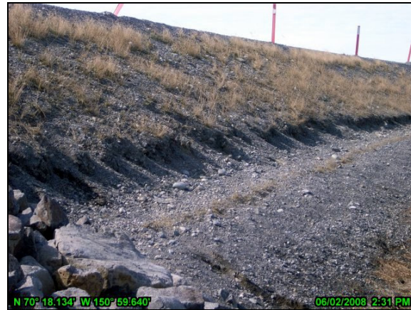
Photo 4-18 CD4 Access Road Fine Grained Sediment Settlement from 2007 Breakup at North Culvert Battery, June 2, 2008
