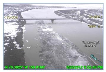
Photo 4.71: Low velocity flow in the Tamayayak moving downstream past the pipe bridge gages, with rafted ice, looking upstream (east); May 25, 2012
