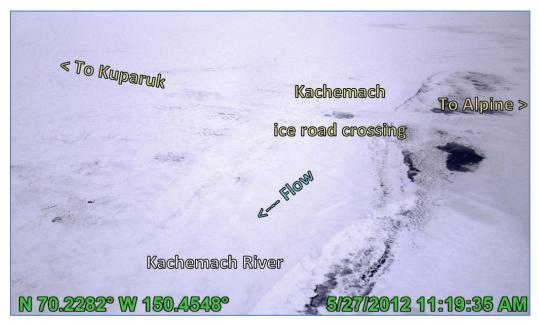
Photo 2.16: Kachemach River ice bridge crossing slotted to facilitate flood flow prior to breakup, looking upstream (south); May 27, 2012
