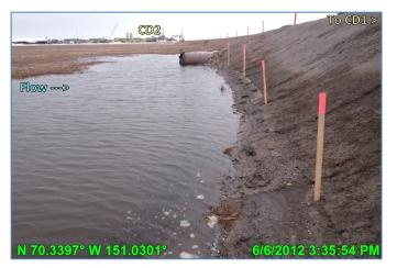
Photo 4.59: Minimal winnowing of fine-grained material on the south side of CD2 road; June 6, 2012
