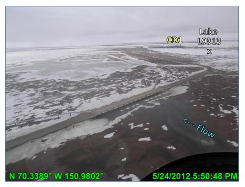
Photo 2.12: View of south side of long swale bridge with snow mechanically removed prior to breakup and local melt in area, looking east; May 24, 2012
