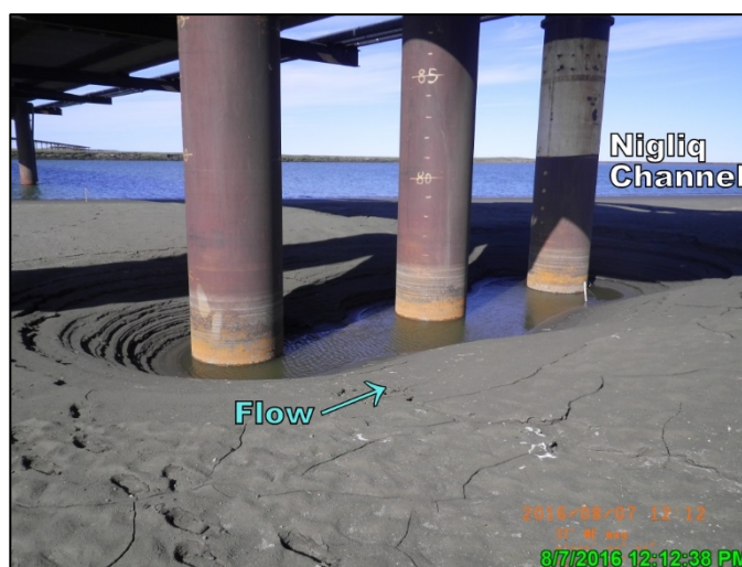
Photo 6.3: Small scour hole around Nigliq Bridge pier 6, piles C, D, & E post-breakup; August 7, 2016
