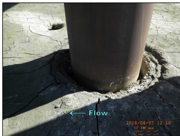
Photo 6.2: Nigliq Bridge pier 8, pile D post-breakup; August 7, 2016
