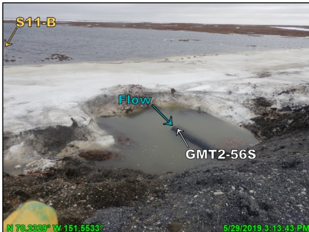
Photo F.10: Blocked culvert GMT2-56 inlet with meltwater ponding, looking south; May 29, 2019
