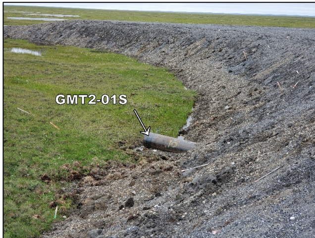
Photo F.22: Extension on culvert GMT2-01, looking west; July 2019
