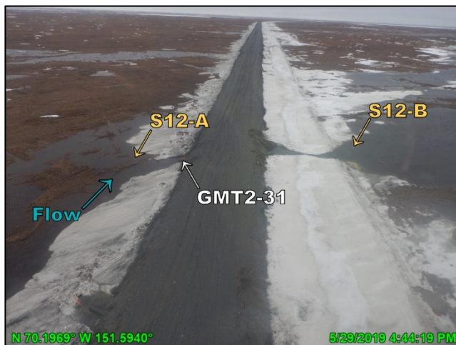
Photo F.20: Minor sloughing near culvert GMT2-31, looking west; May 29, 2019
